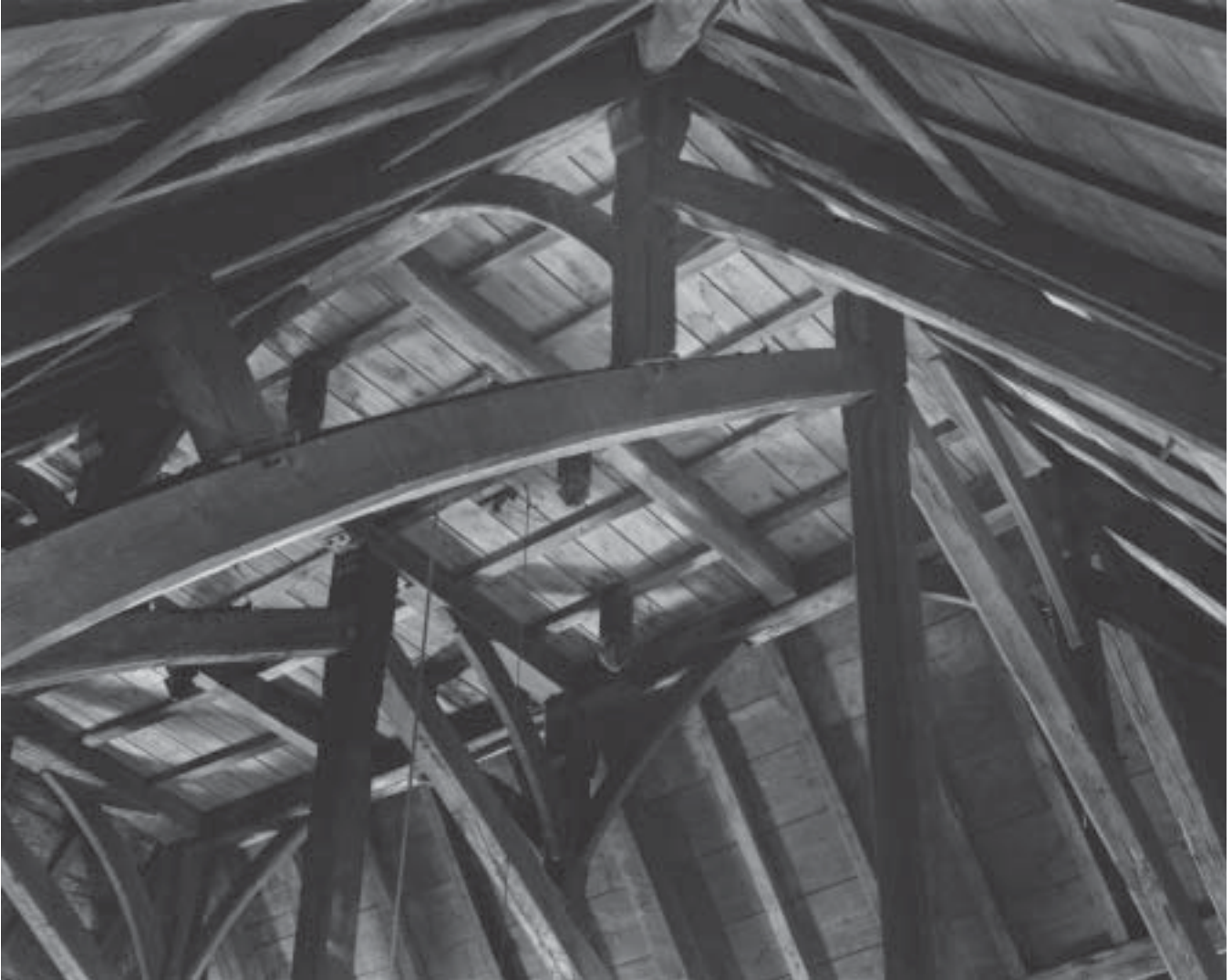
Roof Beams, Old Ship Meetinghouse (1681), Hingham Massachusetts 2008
